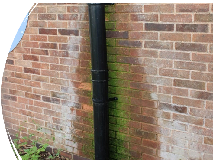
Example damaged rainwater stack pipe that could cause of penetrating damp
