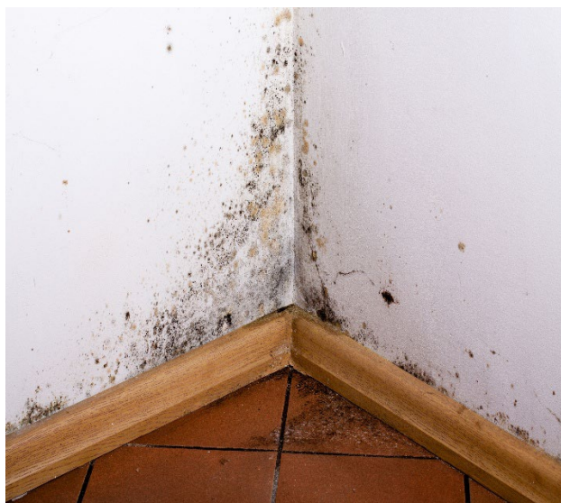
Example of mould related to condensation
