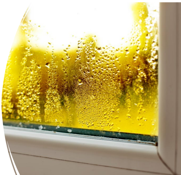
Example of condensation on window pane
