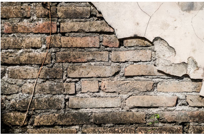
Example external wall and brickwork damage that could cause of penetrating damp
